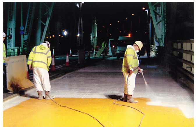
Runcorn Bridge (Courtesy Stirling Lloyd)
