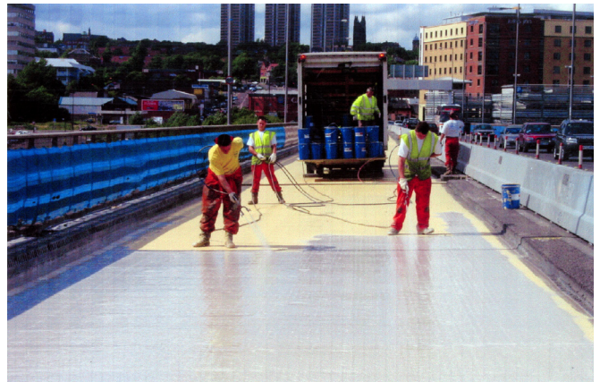
Redhenge Bridge (Courtesy: Universal Sealants (UK) Ltd)
