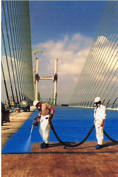
Second Severn Crossing (Courtesy: Pitchmastic)
